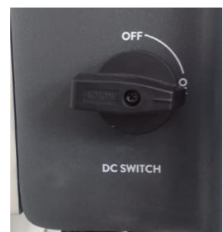
*PV DC switch
